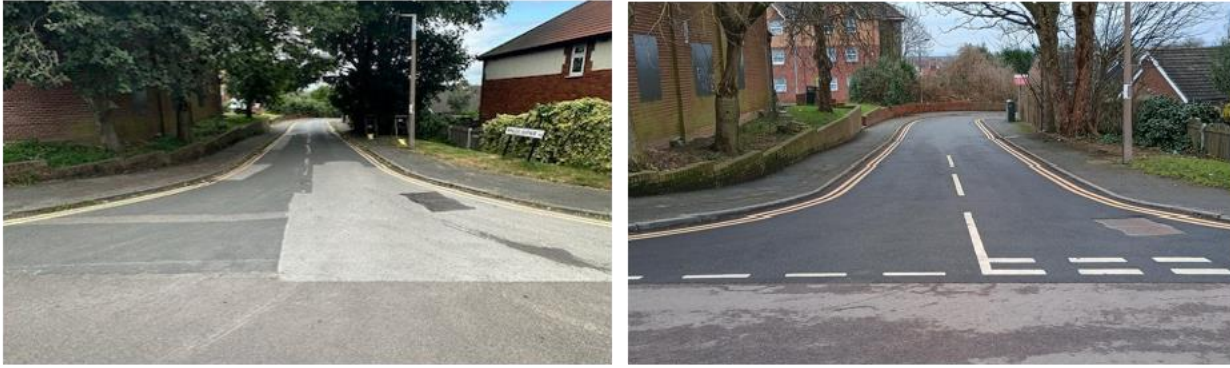
Figure 1 - Winlea Avenue Brecks, Before and After
